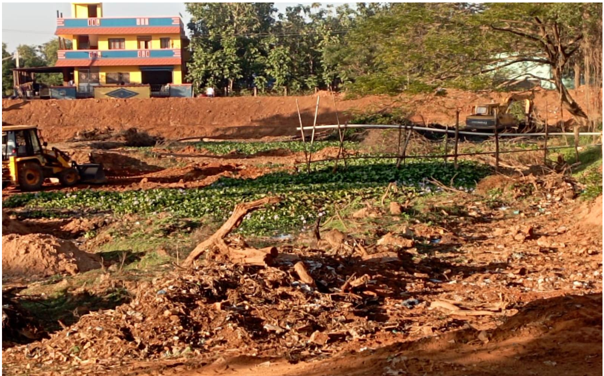
DURING DESILTING WORK
