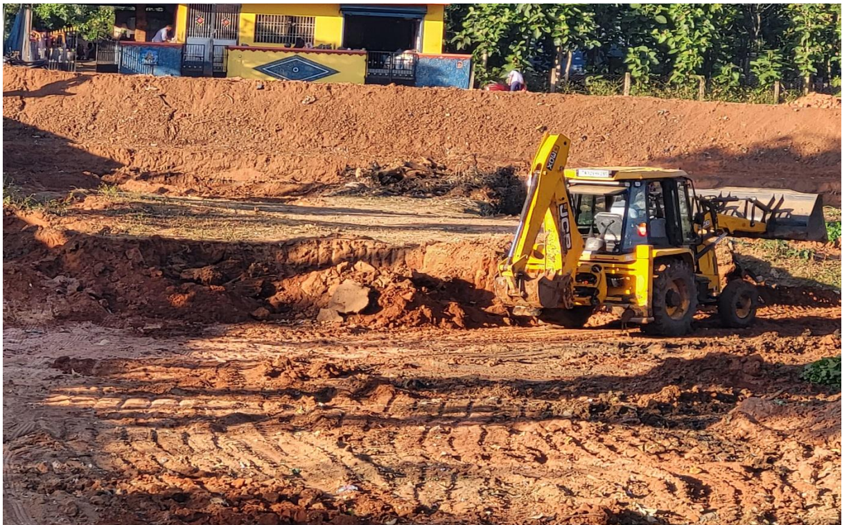
DURING DESILTING WORK
