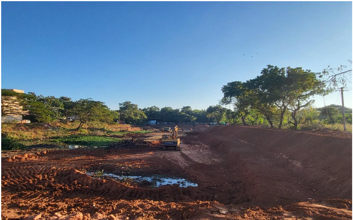
DURING DESILTING WORK
