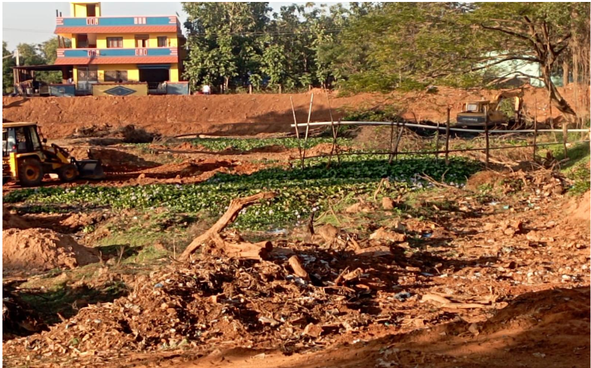
DURING DESILTING WORK
