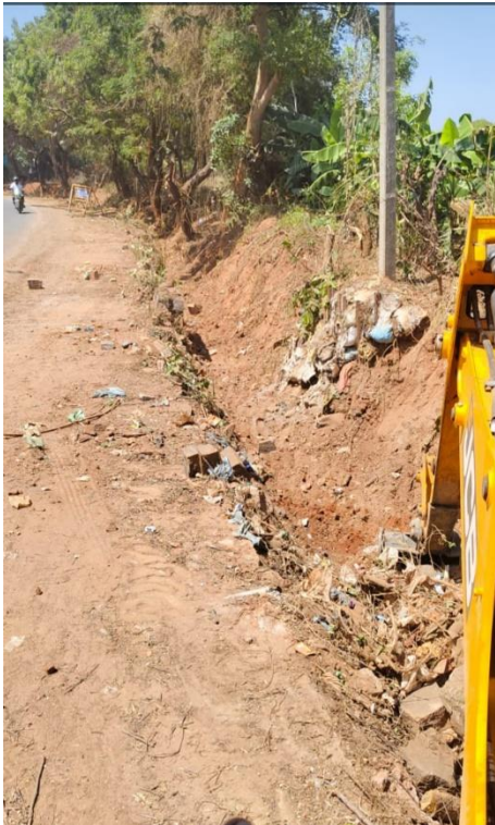
CLEARING THE INLET CHANNEL
