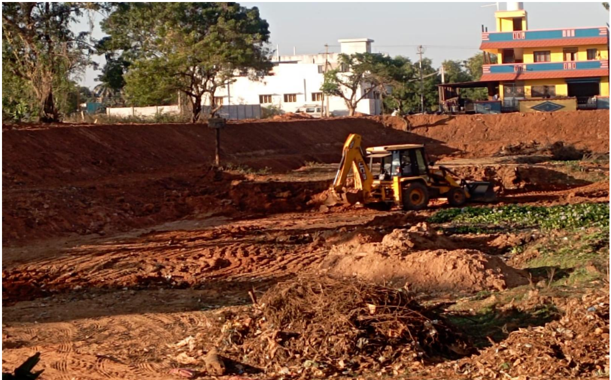
DURING DESILTING WORK
