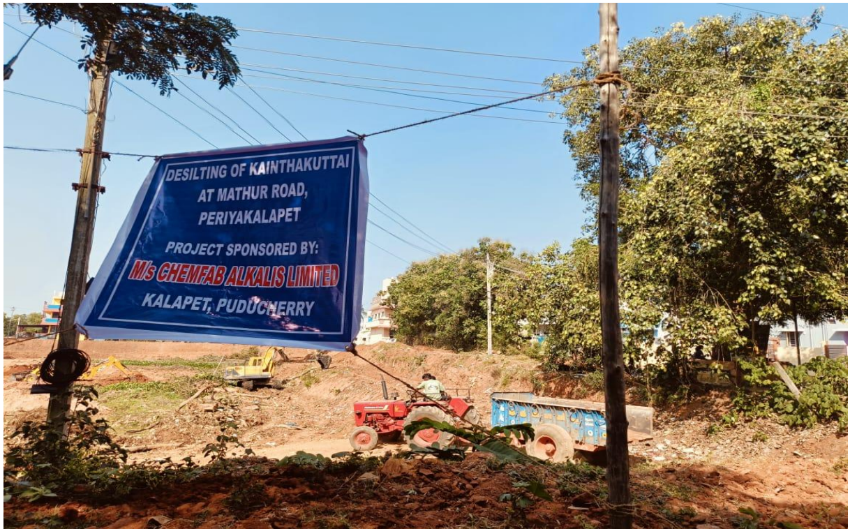
DURING DESILTING WORK
