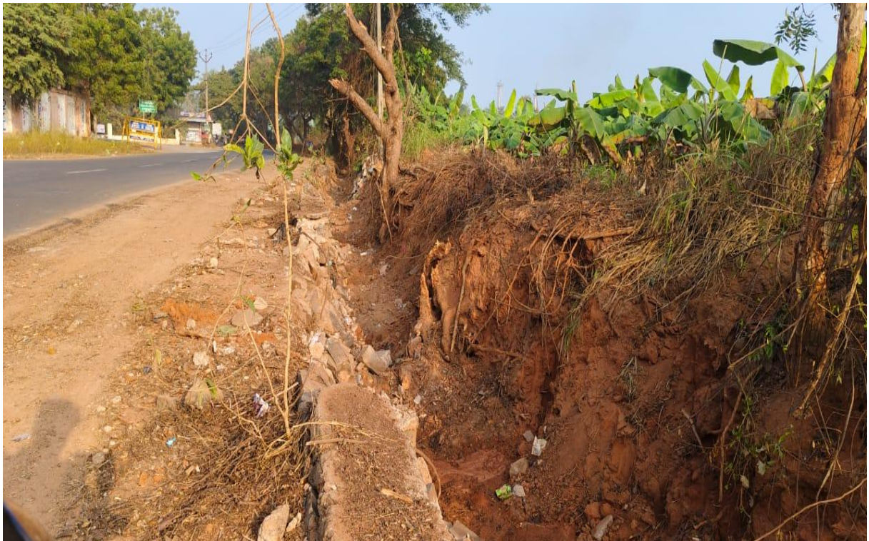
CLEARING THE INLET CHANNEL
